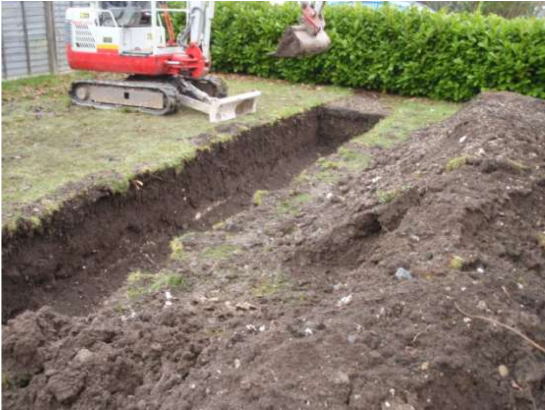
Plate 1. Trench 1 (looking NW)
